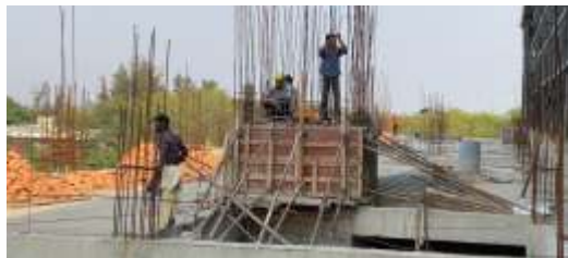
Civil work in progress
