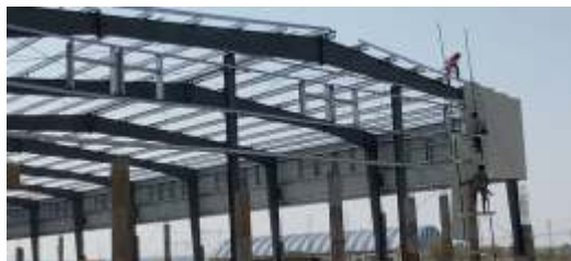
Sheeting work in progress
