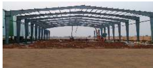
Skeleton Structure Erection
