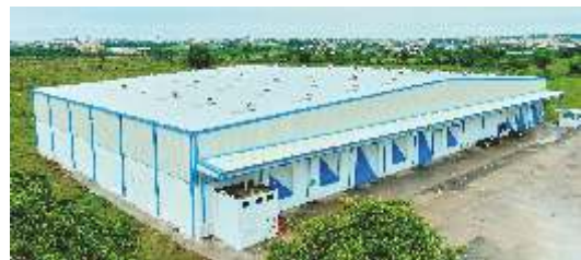
Completed PEB Structure
